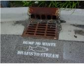
Many people do not realize that the storm water system is separate from the sanitary sewer system. The storm water system collects rain and snow melt
